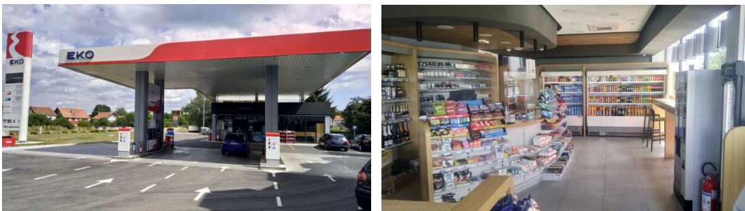
Petrol station Nikšić 3 - after reconstruction
