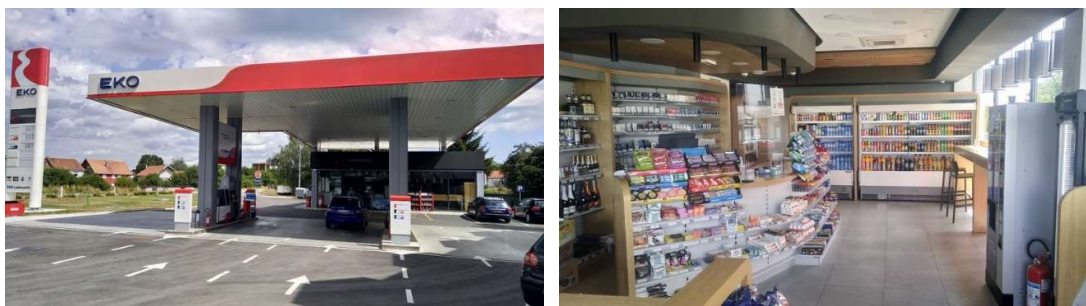
Petrol station Nikšić 3 - after reconstruction
