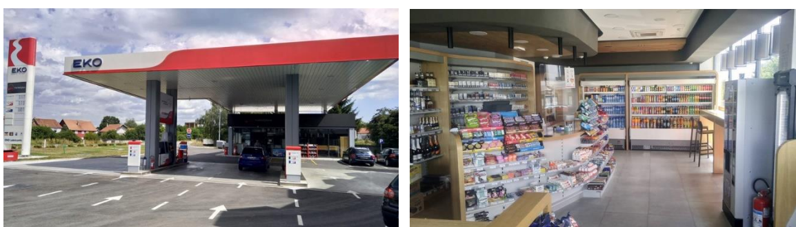
Petrol station Nikšić 3 - after reconstruction
