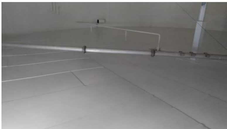
Anticorrosive protection of pipelines and tanks
