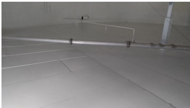
Antocorrosive protection of pipelines and tanks
