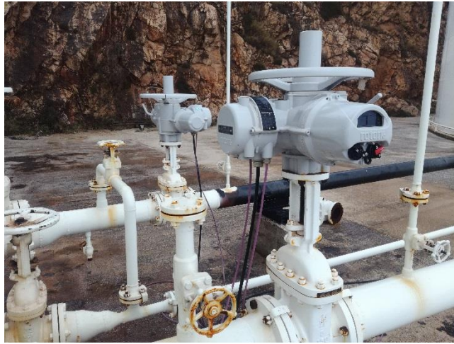
Installed MOVs at inlet and outlet tank pipelines
