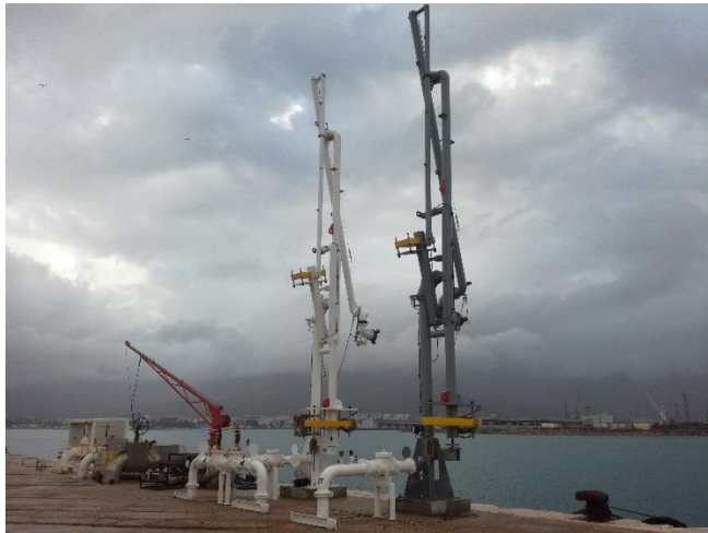
Installed four new marine unloading arms
