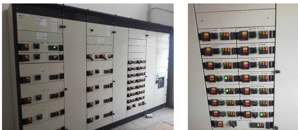
New switchboards for pump and other facilities management
