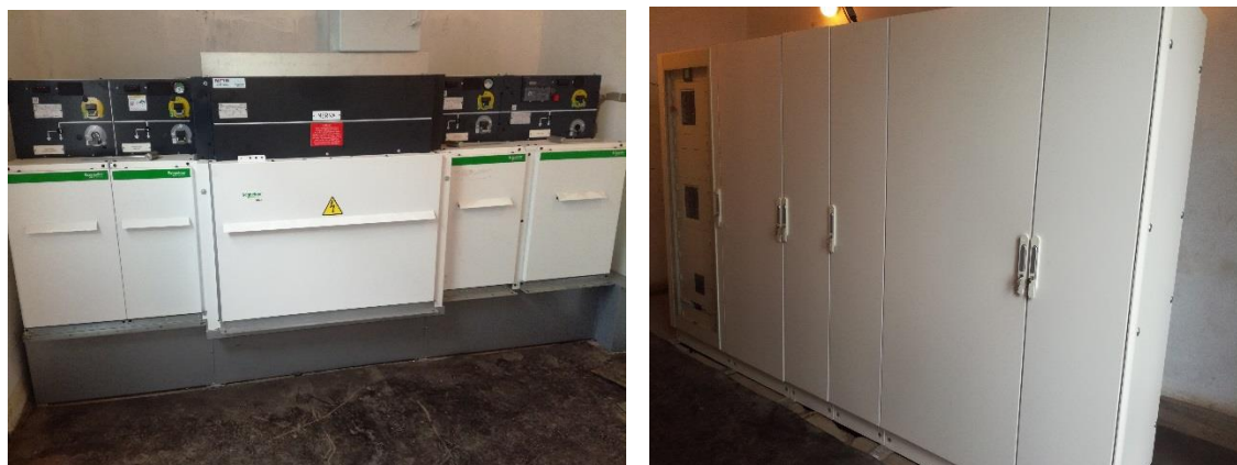
Reconstruction of substations: new 10 kV and 400 V segments
