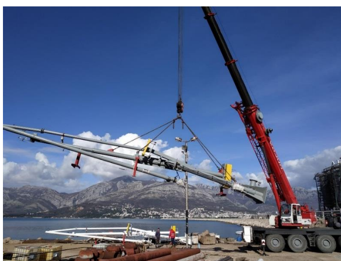
Marine unloading arms at factory premises and unloading at bar Terminal
